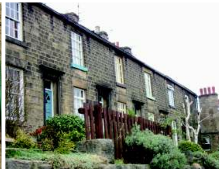
Picture 46 Terraces along Reservoir Road
