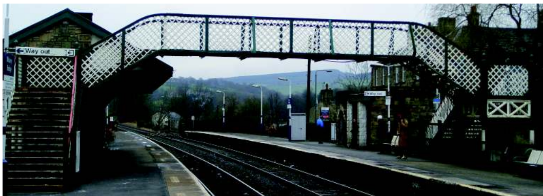
Picture 34 The cast iron footbridge that spans the railtrack
