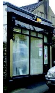
Picture 31 Shop front at 1 Bridge Street
