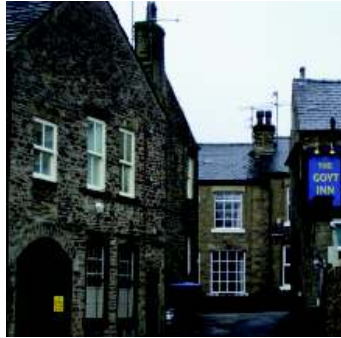
Picture 30 View from Chapel Street towards Bridge Street
