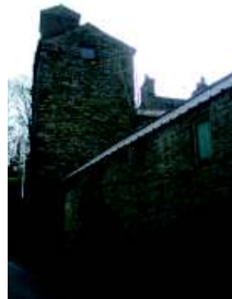
Picture 56 The disused colliery air shaft at the start of Bings Road
