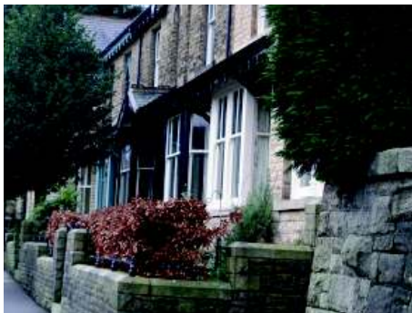
Picture 47 21 - 25 Reservoir Road - a particularly well preserved row of buildings
