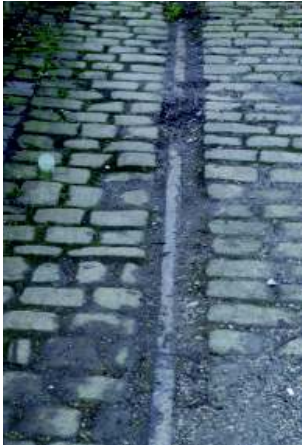
Picture 23 Visible railway tracks along Bingswood Avenue
