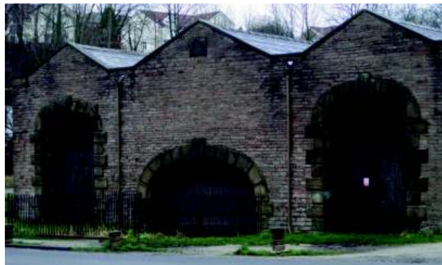
Picture 22 Front elevation of the warehouse building
