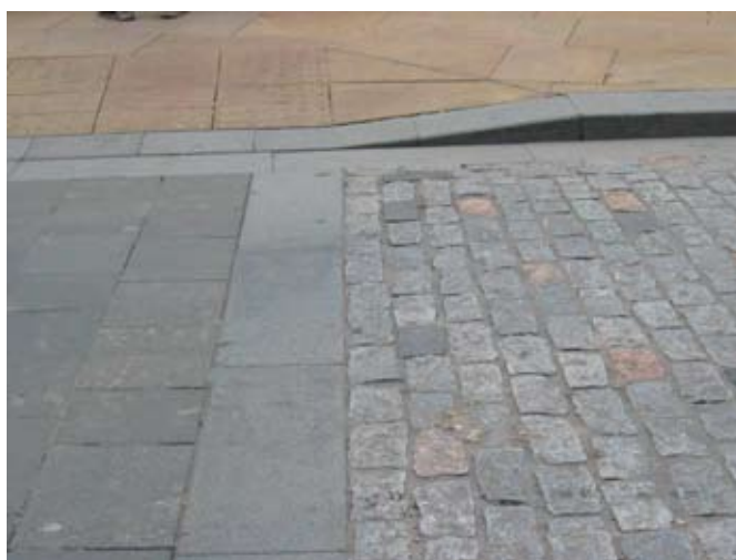
Natural Stone Paving in Footpath and Carriageway
