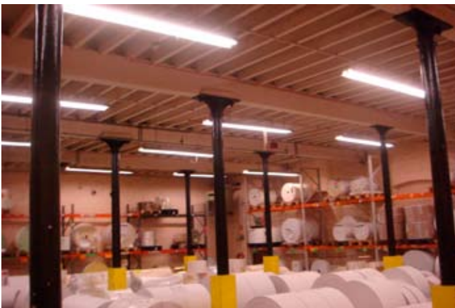
Floor space broken up by cast iron columns
